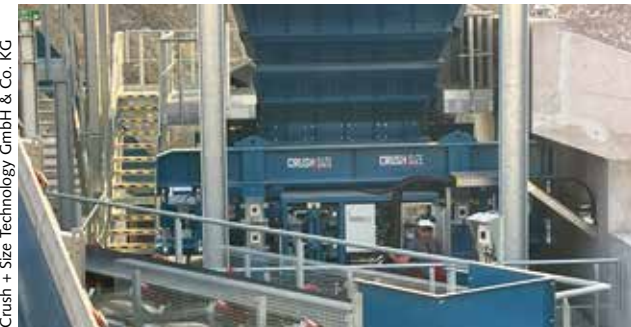
Installation Primary Crusher DRC 900-20
